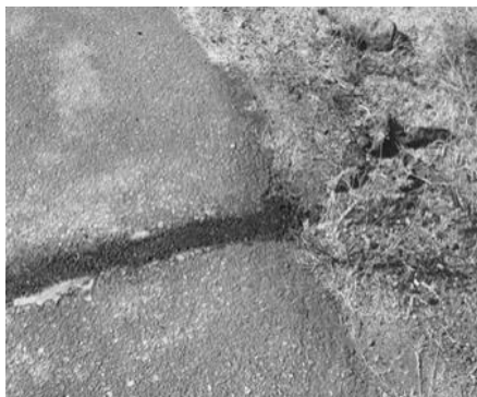
Bay Trail crack repaired with slag in shoulder
