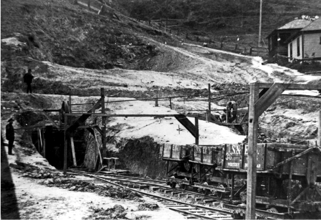
Above: Three holes were drilled and the core between them removed. Considerable trouble was experienced due to cave ins which delayed the completion date (0053-DC from Don Church)
