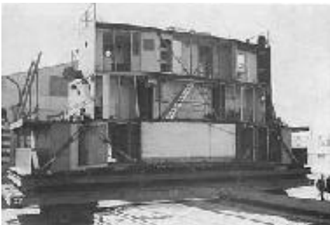
A deckhouse section is moved into position to be lifted by Whirley cranes onto ship. Fully furnished, it has look of a cutaway stage set. To best judge scale, note the two figures in corner, lower right.
