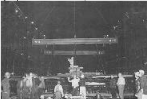
Midnight 11/08/42 work begins. The keel of the Peary is carefully lowered onto the shipway.
