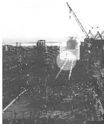
Only moments after Peary launching, keel for next ship (inside highlighted circle) is lowered into position.
