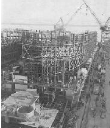
Early on first day, the hull is already rising up off the shipway
